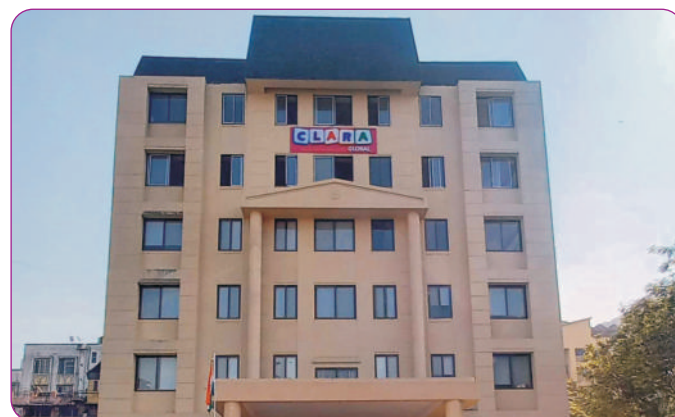
New School Building
